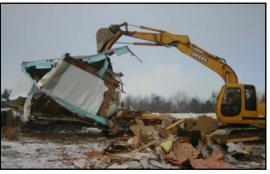
was removed the coinciding sections of wall was broken into the middle of the structure. A significant amount of the home contained mold and rotting wood, which slowed down the deconstruction process. In addition to metal components, a stove and water tank were sorted from the waste pile and appropriately recycled. This mobile home's weight was
