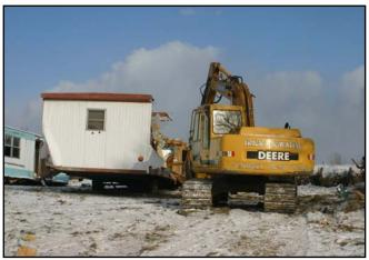
the remnants of the walls were crushed into the center of the structure. The metal and waste were then separated into two piles and the remaining frame was chopped into pieces and placed in the metal pile.
